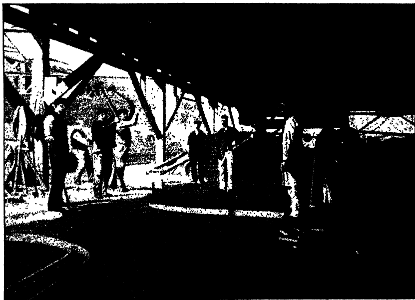
BENDING FRAMES FOR TURRET VESSEL.
